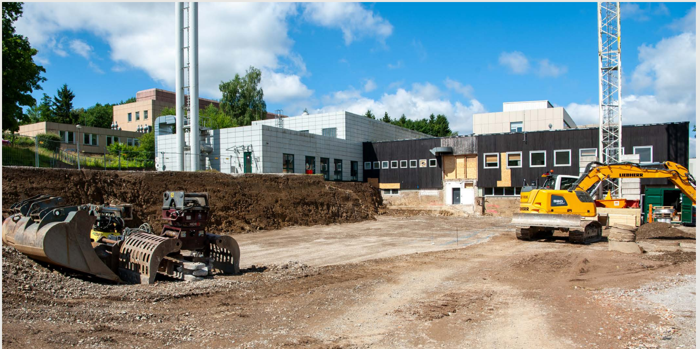
Baustart am Clausthaler Chemie Campus.
